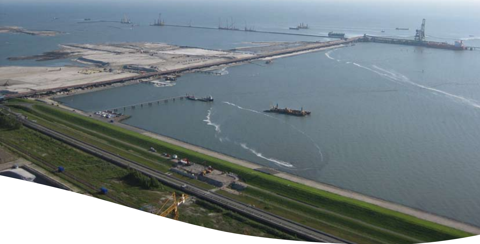
Cooling water intake site
